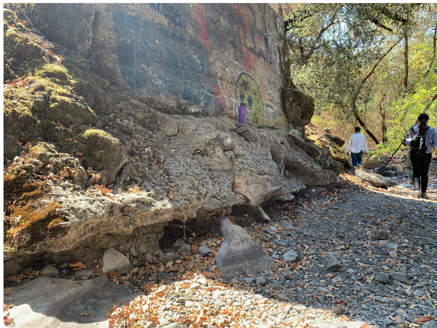
Photo 1 – Southern abutment (looking southwest)
