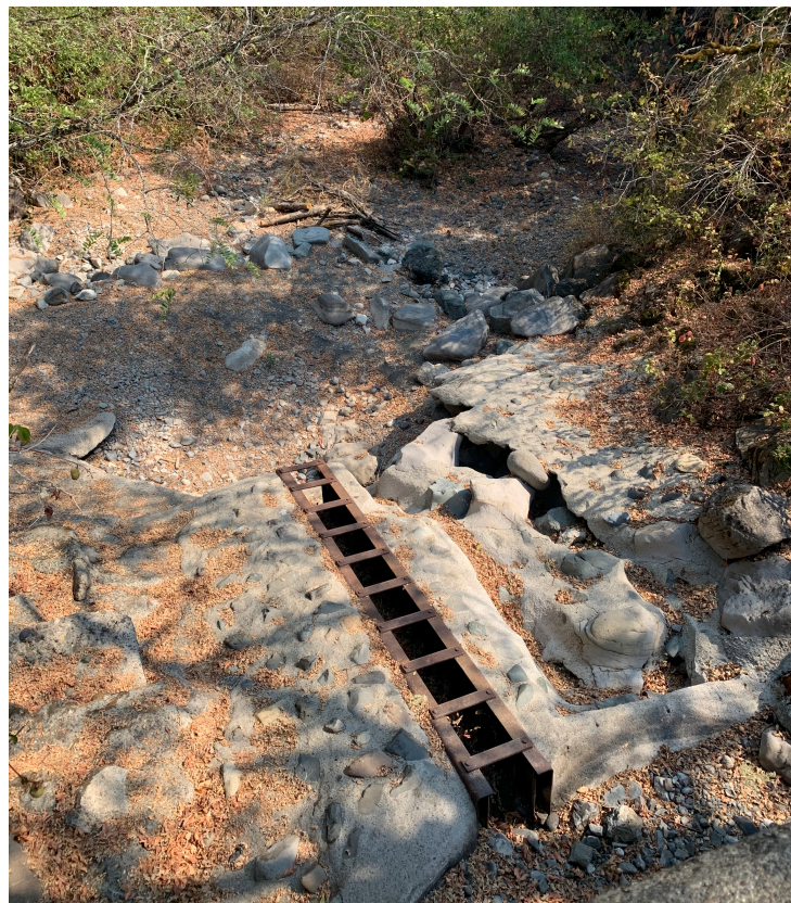
Photo 3b – Fish ladder/rock weir (looking east)
