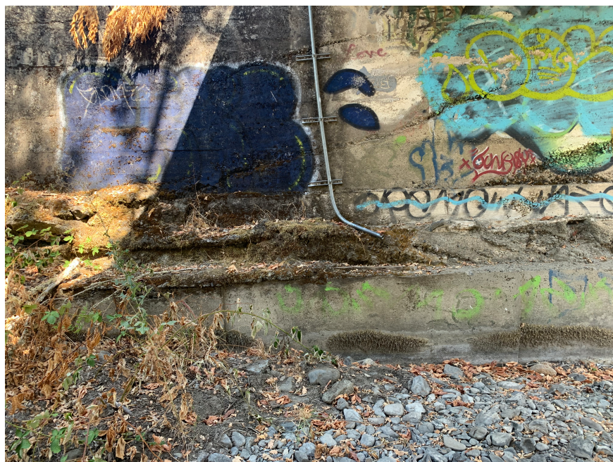
Photo 2 – Northern abutment (looking north)
