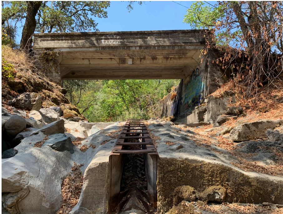
Photo 3a – Fish ladder (looking west)
