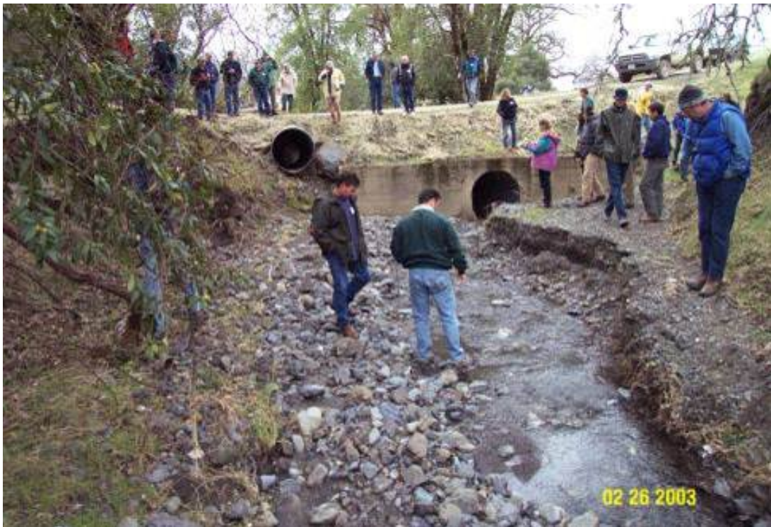
Figure 1. Example of a critical culvert installed at a stream crossing with diversion potential (Pacific Watershed Associates Inc. 2003).
