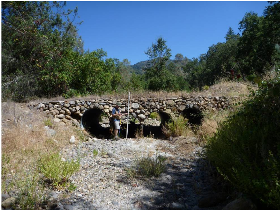
4.6d. Four barrel culvert crossing on Garnett Creek. 8/29/11
