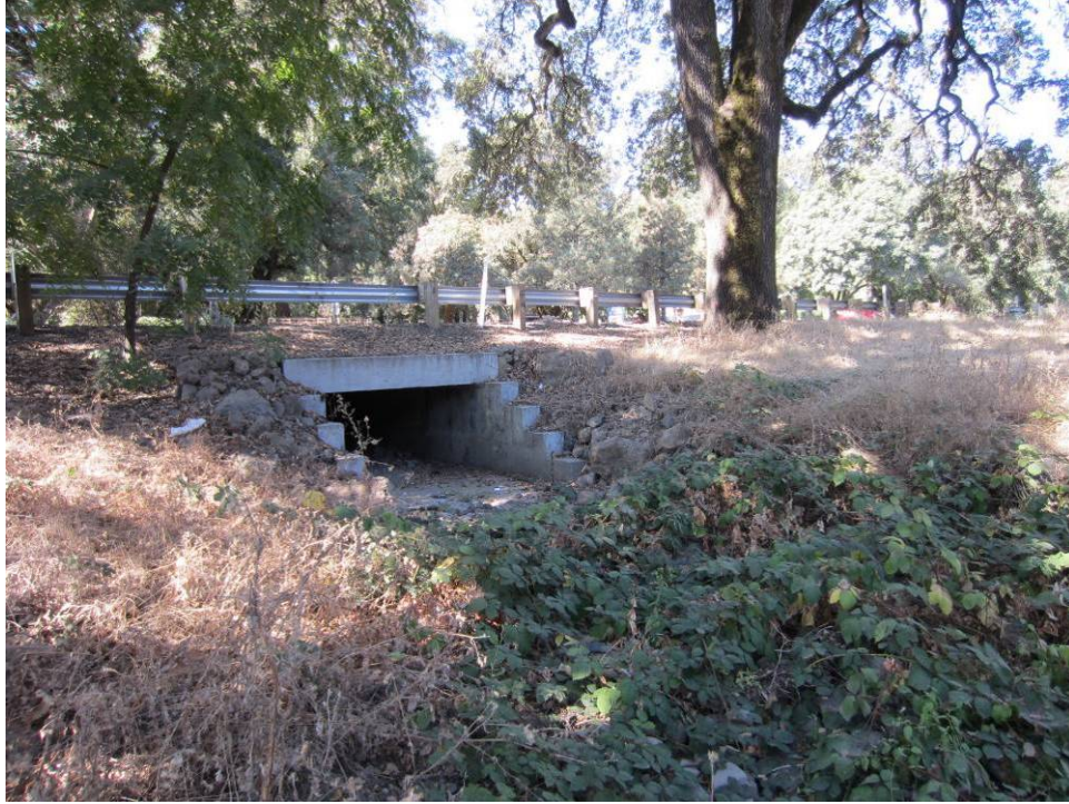
4.3c. Culvert crossing under Highway 29. 9/29/11
