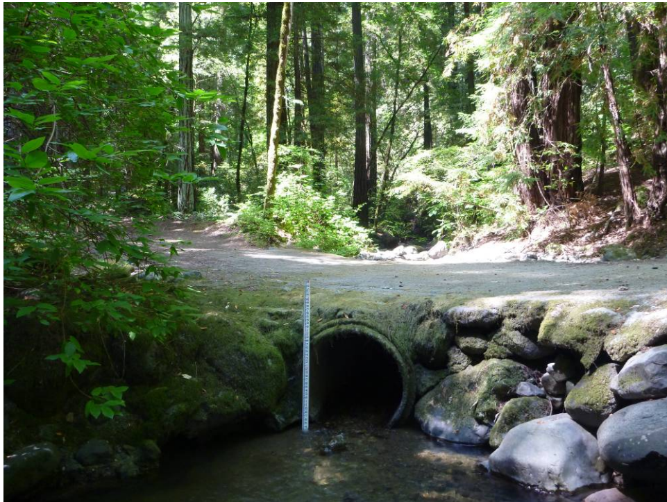
4.2h. Culvert crossing under dirt road within Bothe-Napa Valley State Park. 8/11/11
