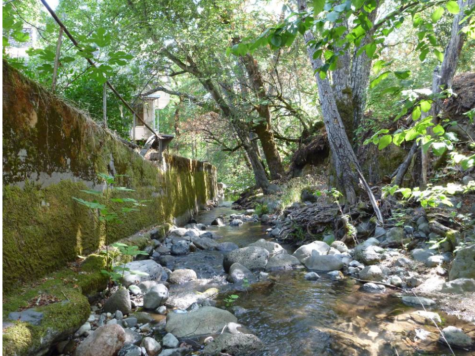
4.2c. Remnants of the diversion dam removed in 2003. 8/10/11
