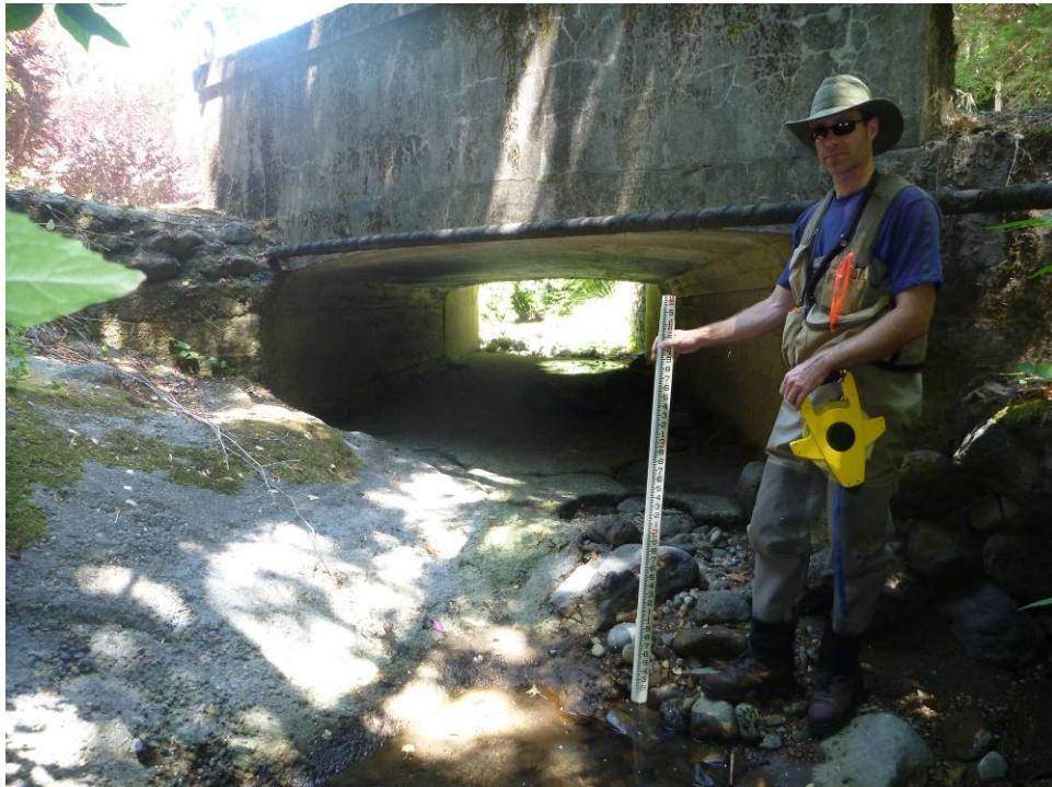
4.4f. Culvert crossing under Diamond Mountain Road. 8/16/11
