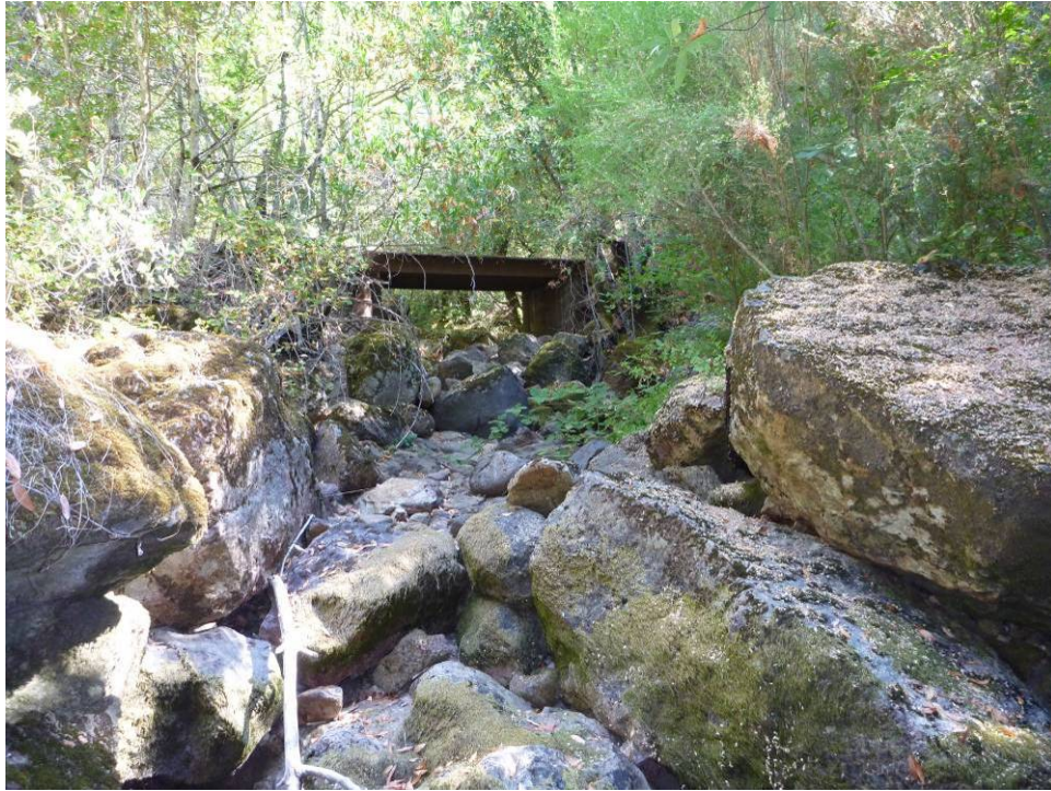
4.6k. Horns Creek with characteristic dry stream bed and steep boulder cascade. 8/31/11
