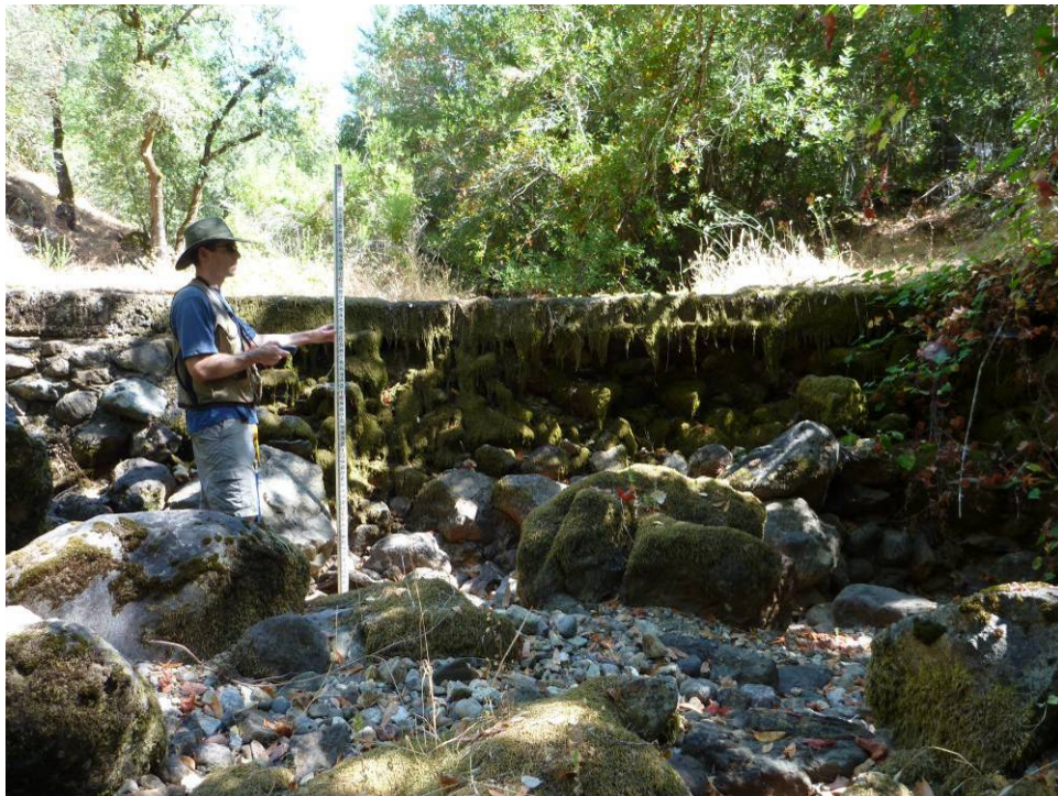
4.6j. Concrete road crossing on Hoisting Works Canyon Creek. 8/29/11
