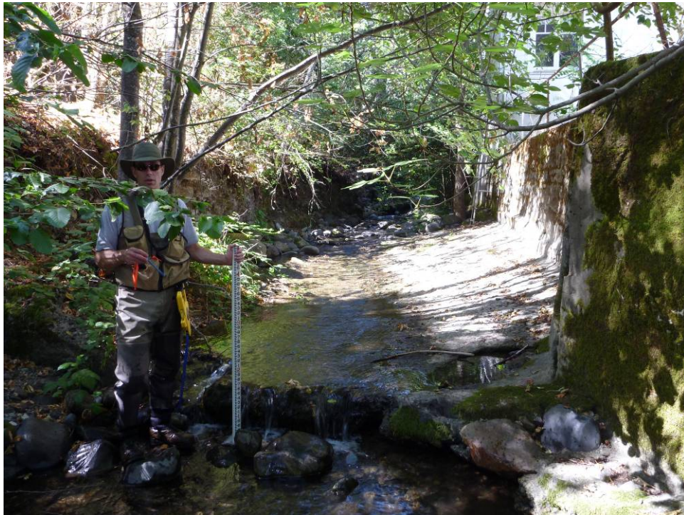
4.2d. Remnants of the diversion dam removed in 2003. 8/10/11
