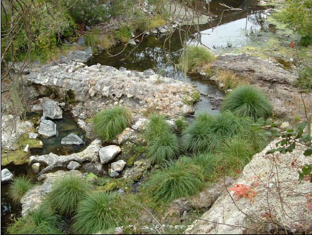
Figure 9. Downstream step-pool sequence and grouted rock weir, looking upstream.
