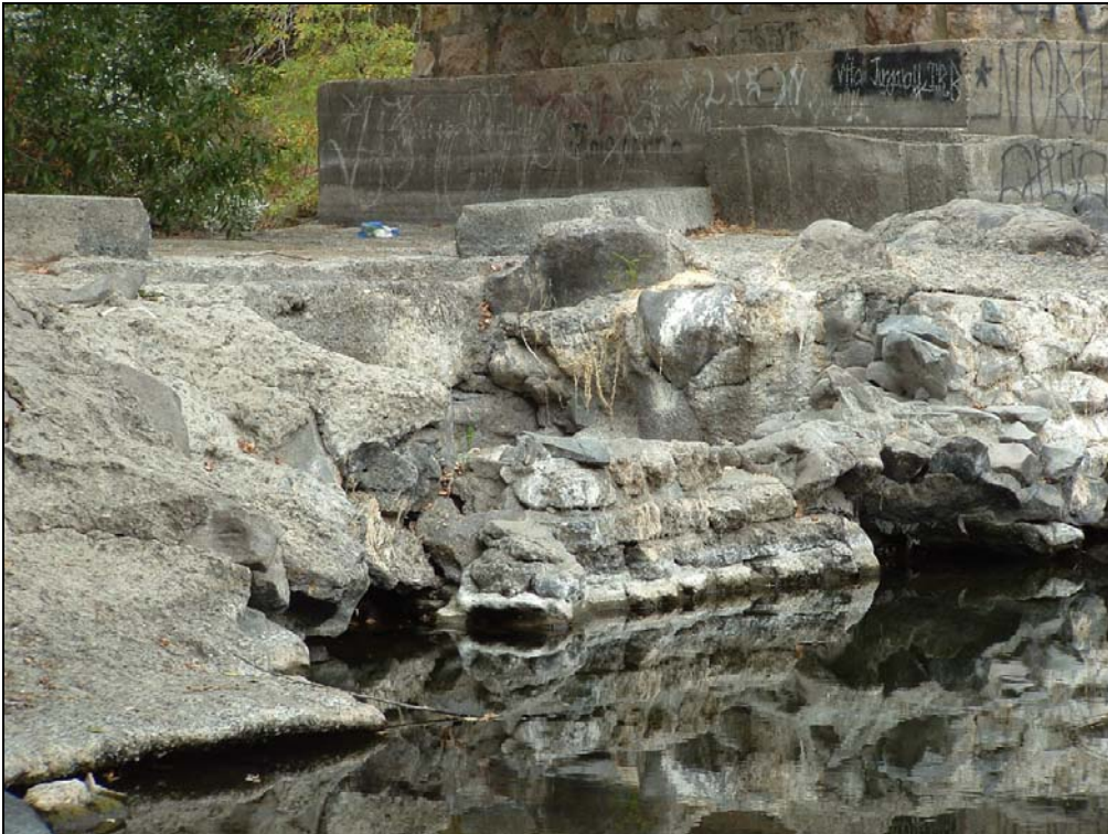
Figure 3. Western bridge opening, looking upstream
