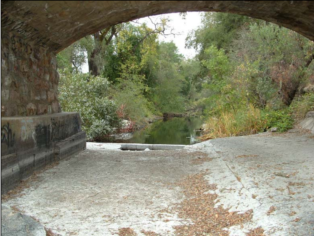
Figure 4. Eastern bridge opening, looking upstream.
