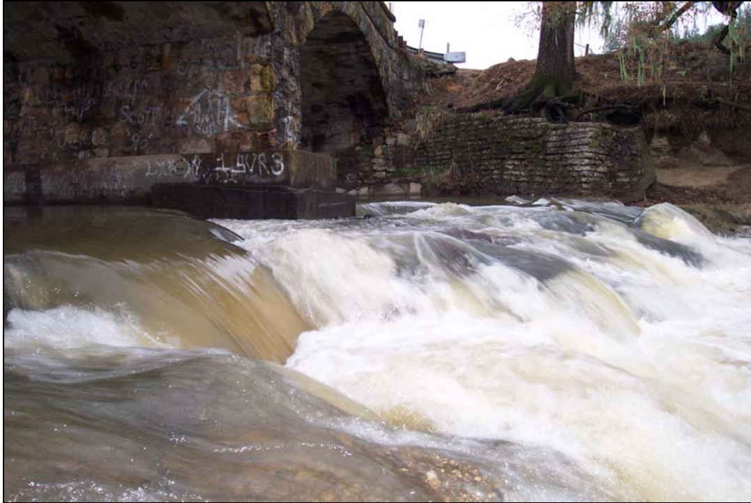
Zinfandel Lane Bridge facing east (12-20-05)
