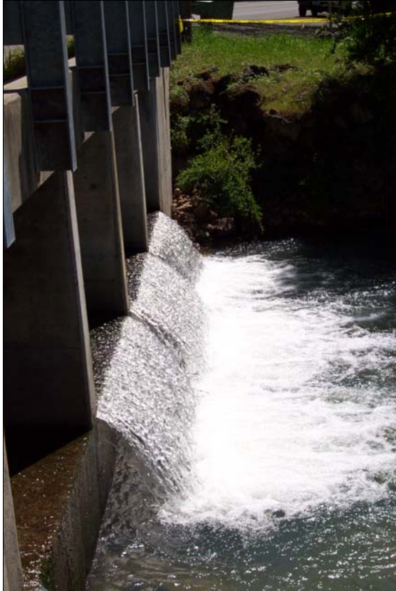
Silverado Trail culvert downstream standing right bank (3-10-2006)
