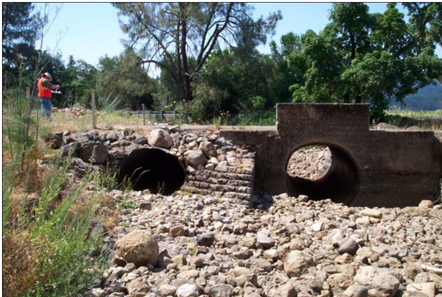
Dutch Henry Culvert inlet facing downstream (5-17-2006)
