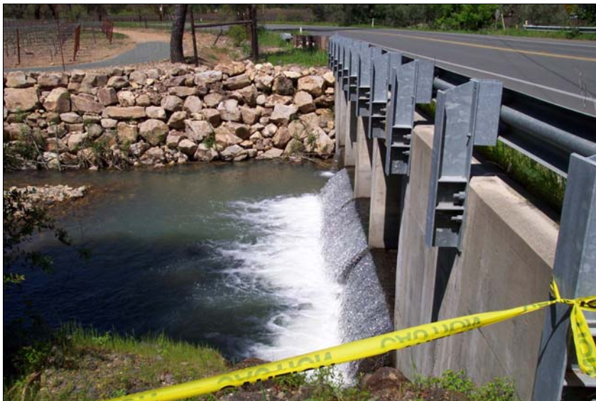
Silverado Trail culvert downstream standing on left bank (3-10-2006)
