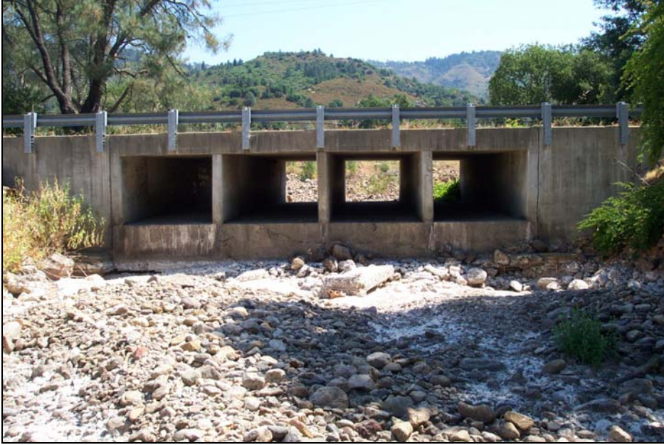
Silverado Trail culvert facing upstream (5-17-2006)
