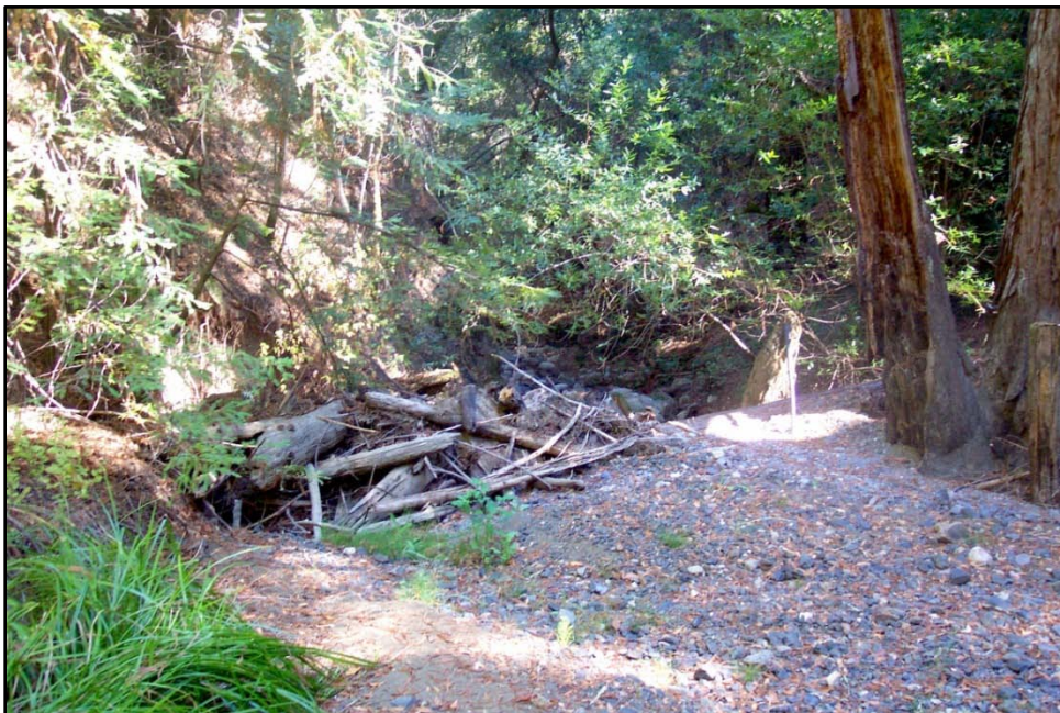
Figure 3. Looking downstream from the earthen ford under summer flow conditions prior to clearing of the debris jam.
