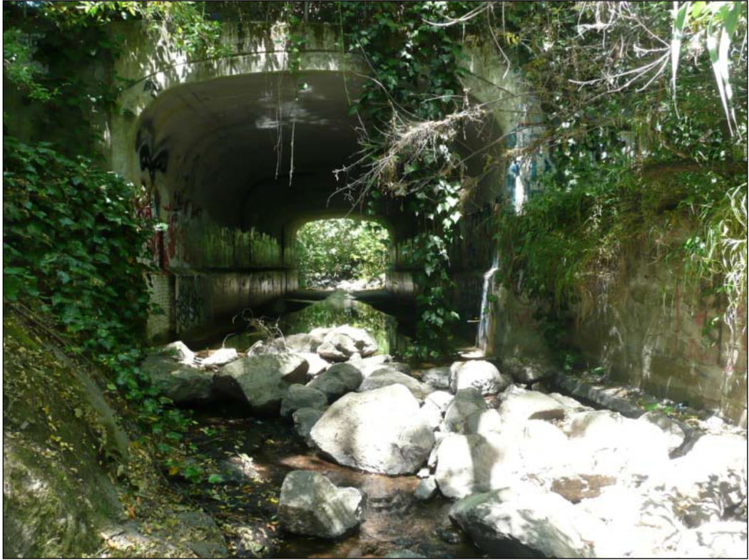
Figure 4. View of downstream face of culvert looking upstream.
