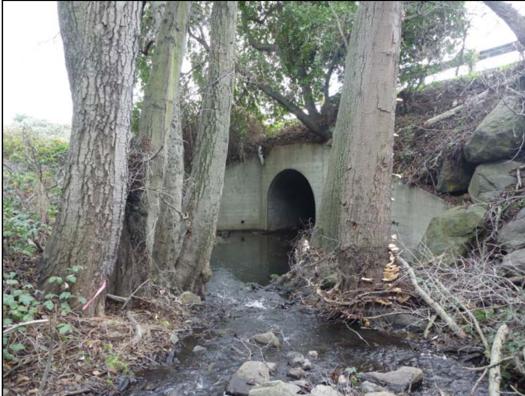
Figure 2. View of upstream culvert inlet and wing-walls looking downstream.
