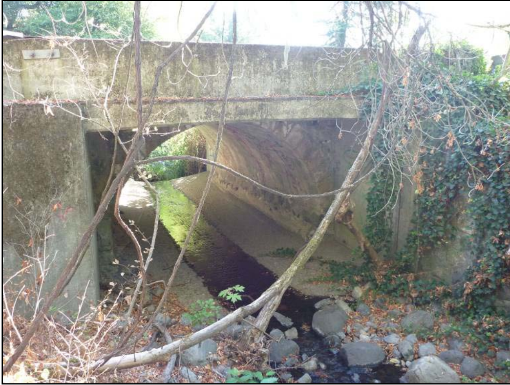
Figure 2. View of upstream culvert face looking downstream.
