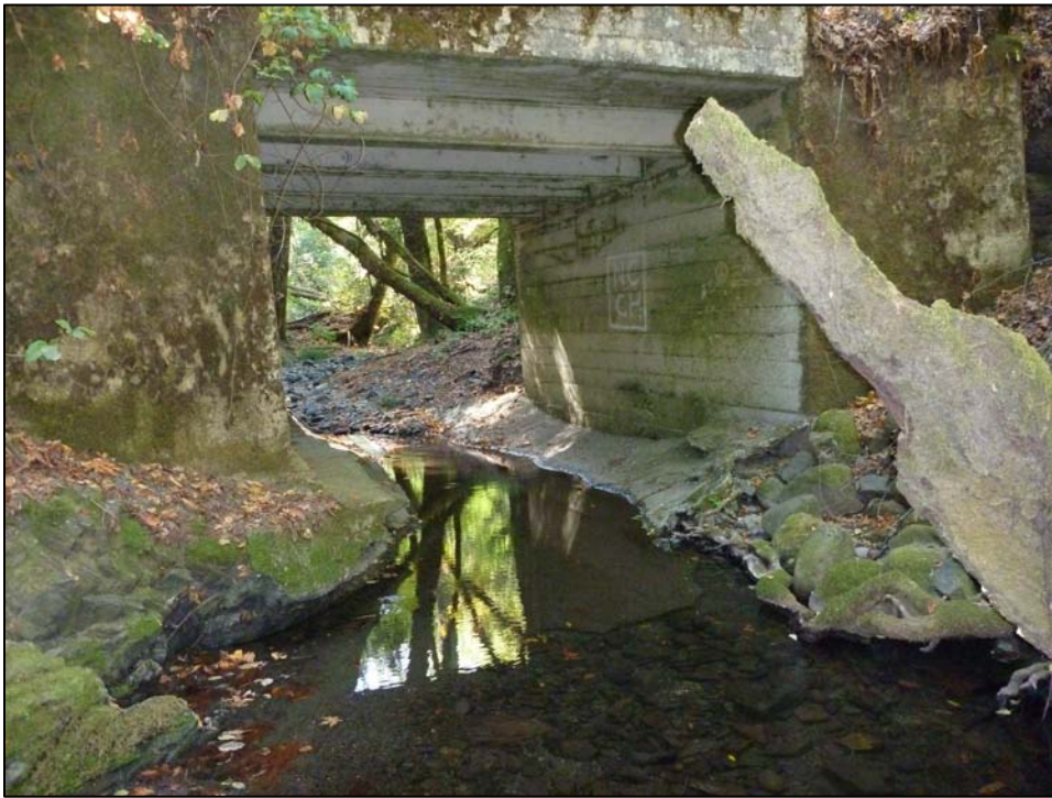
Figure 10. Sulphur Creek culvert at Sulphur Springs Road
