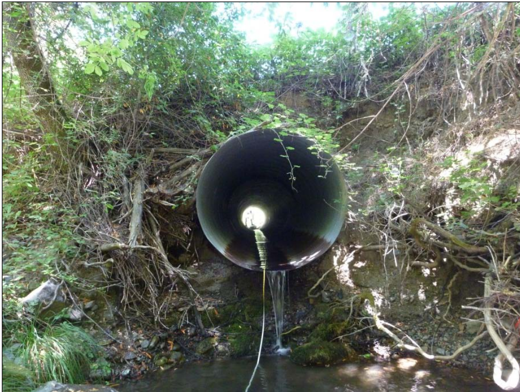
Figure 3. View looking upstream through the Dry Creek Road culvert.
