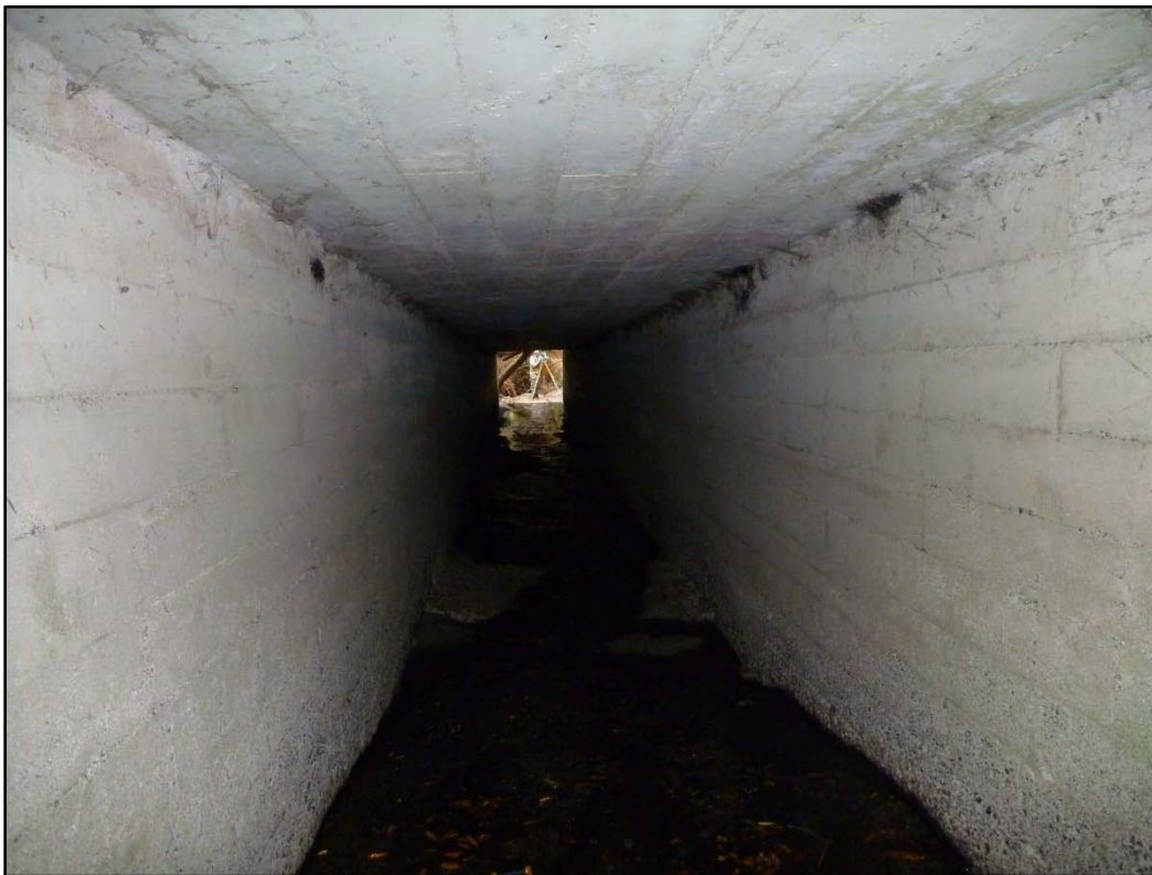
Figure 3. Looking downstream through the culvert.
