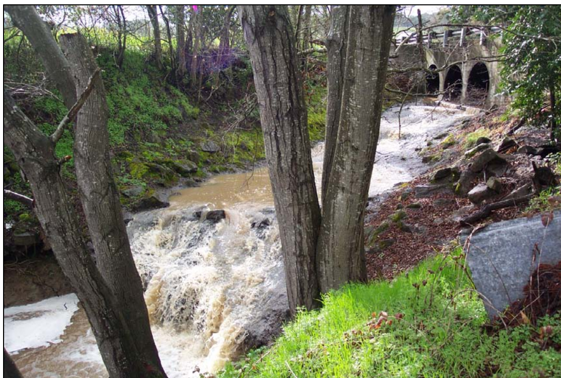
Figure 8. Huichica Creek culvert at Highway 12/121.
