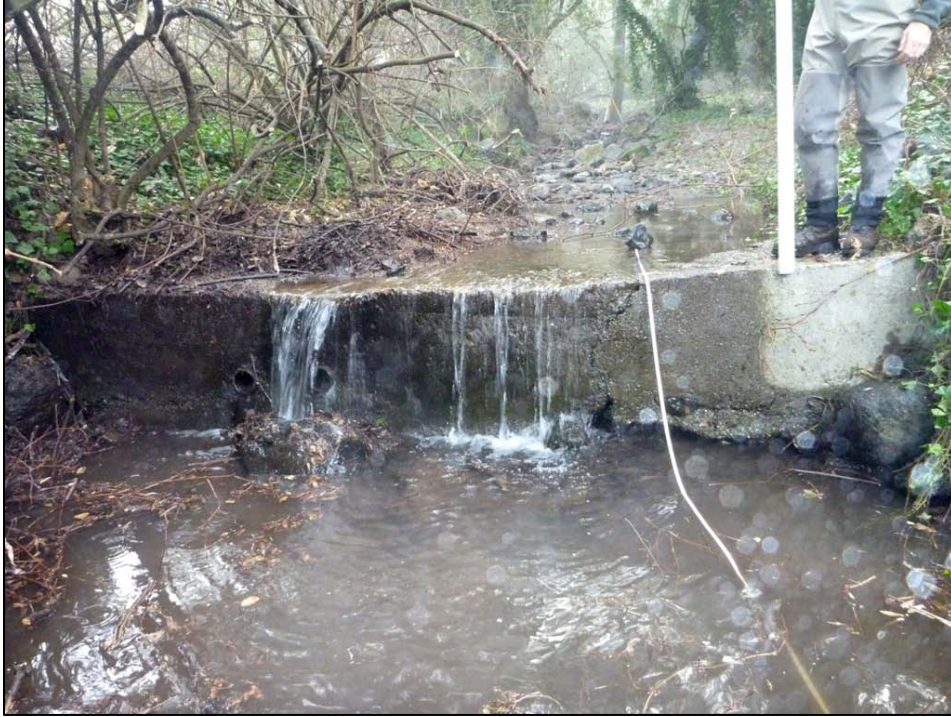
Figure 4. Closer view of the concrete weir at site MUR-3.
