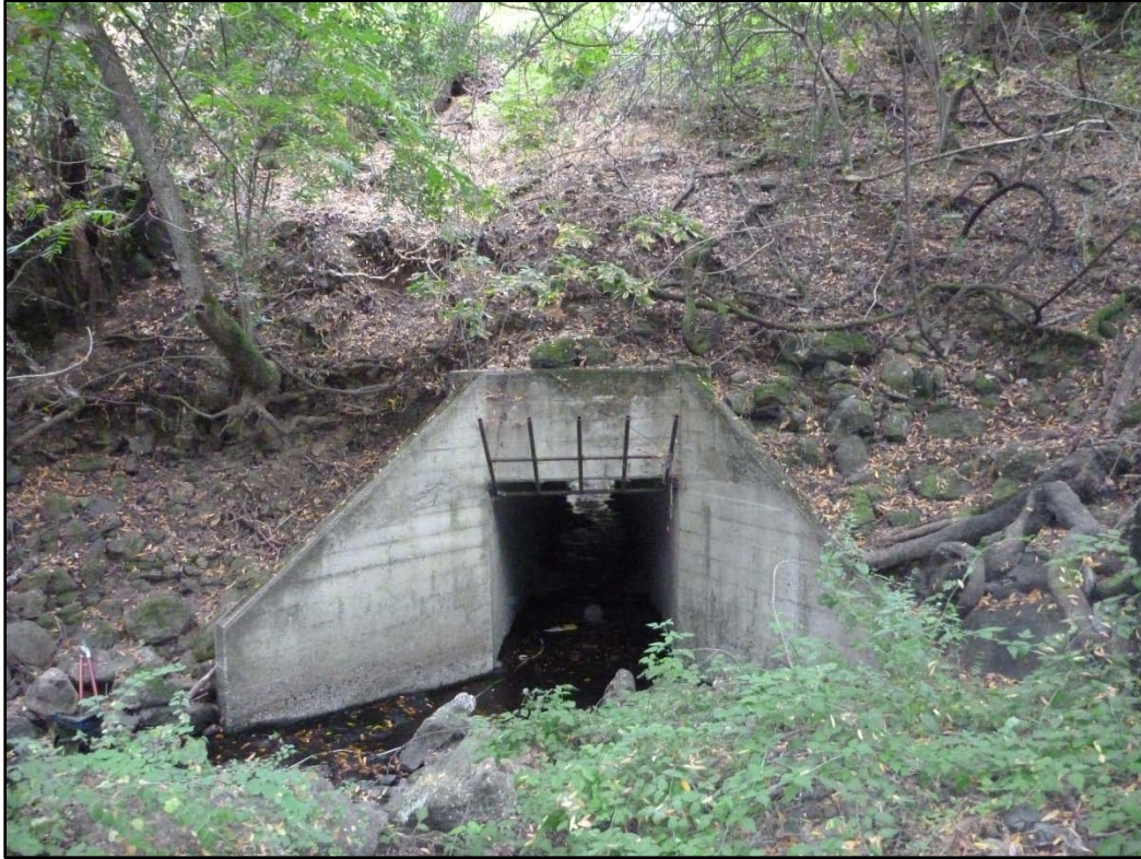
Figure 2. View of culvert inlet looking downstream.
