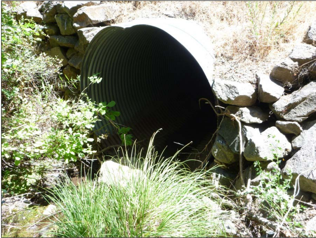
Figure 2. View of the inlet of the Dry Creek Road culvert.
