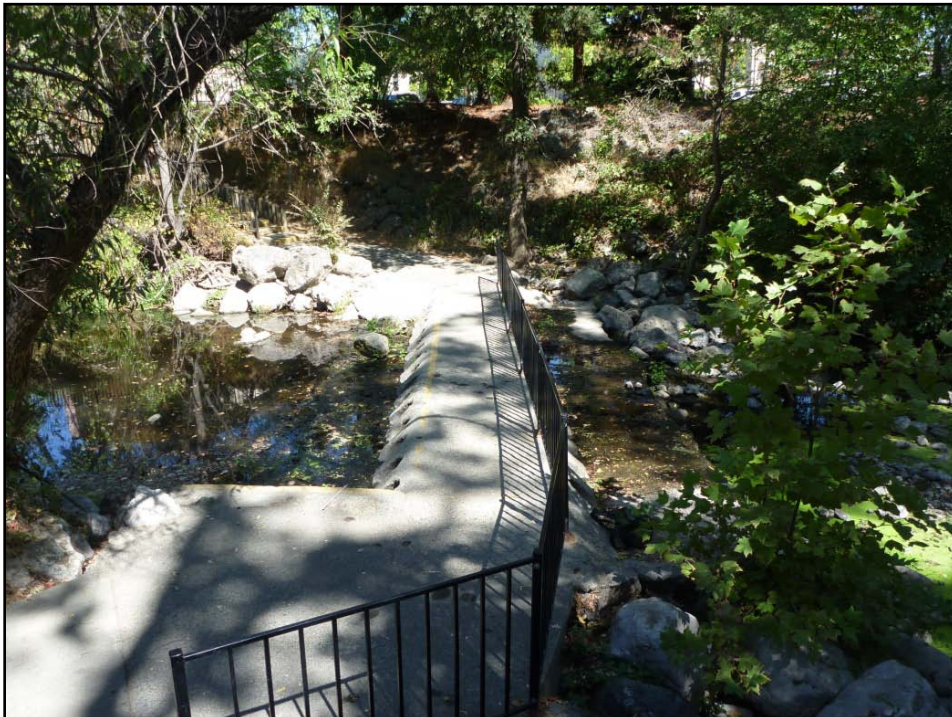
Figure 3. View of foot path from the west bank looking east. Note: seasonal railing is installed on downstream side.
