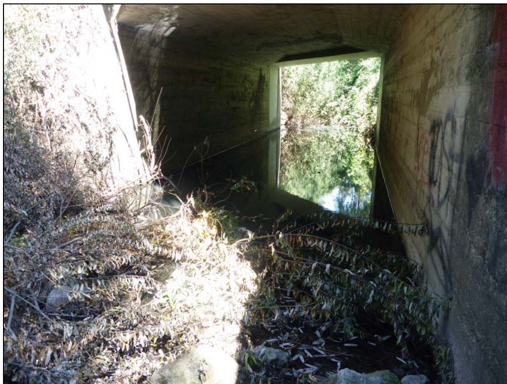
Figure 7. Bell Creek culvert at the Silverado Trail (facing upstream)
