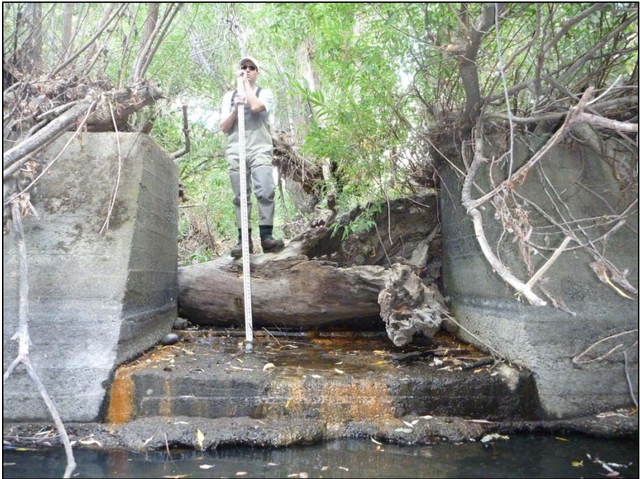
Figure 4. Looking upstream at the lower water channel and jammed log under summer zero-flow conditions.
