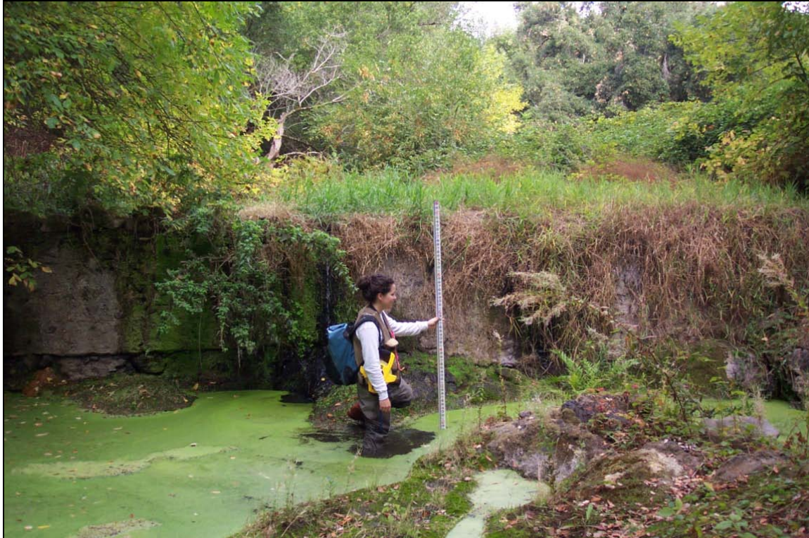
Figure 3. Looking upstream at the dam face under zero-flow conditions.
