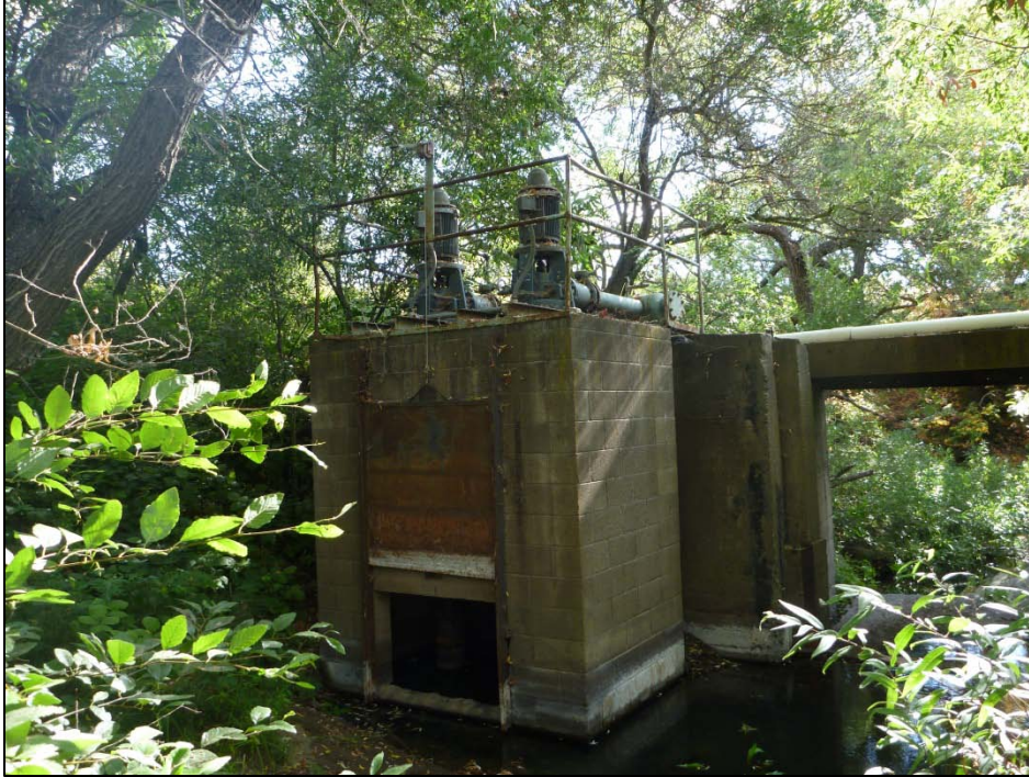
Figure 5. Looking downstream at the pump house and left bank bridge abutment.
