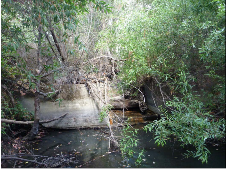
Figure 3. Looking upstream at the defunct flashboard dam under summer zero-flow conditions.
