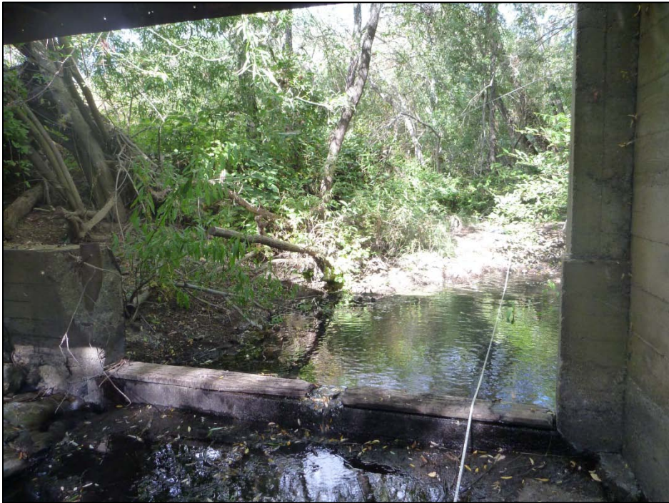
Figure 4. Looking upstream at the weir under summer low flow conditions.
