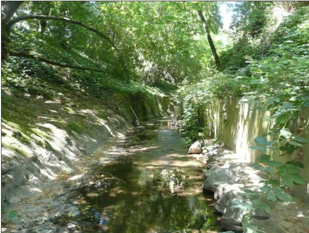
Figure 5. View looking upstream toward culvert from downstream end of concrete apron.
