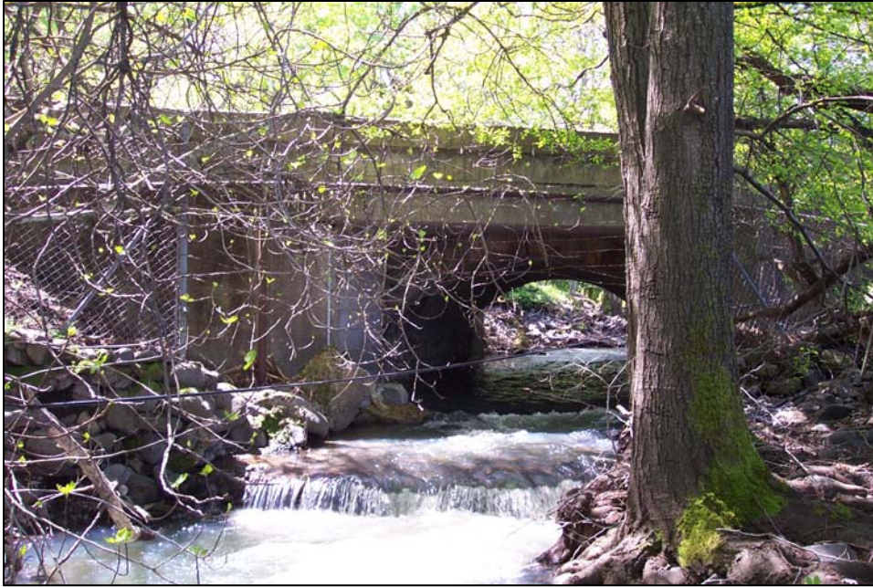
Figure 9. Ritchey Creek culvert at Highway 29
