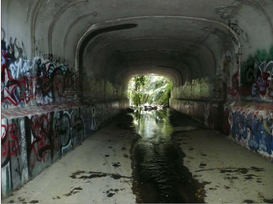
Figure 3. Looking downstream through the Robinson Lane culvert.
