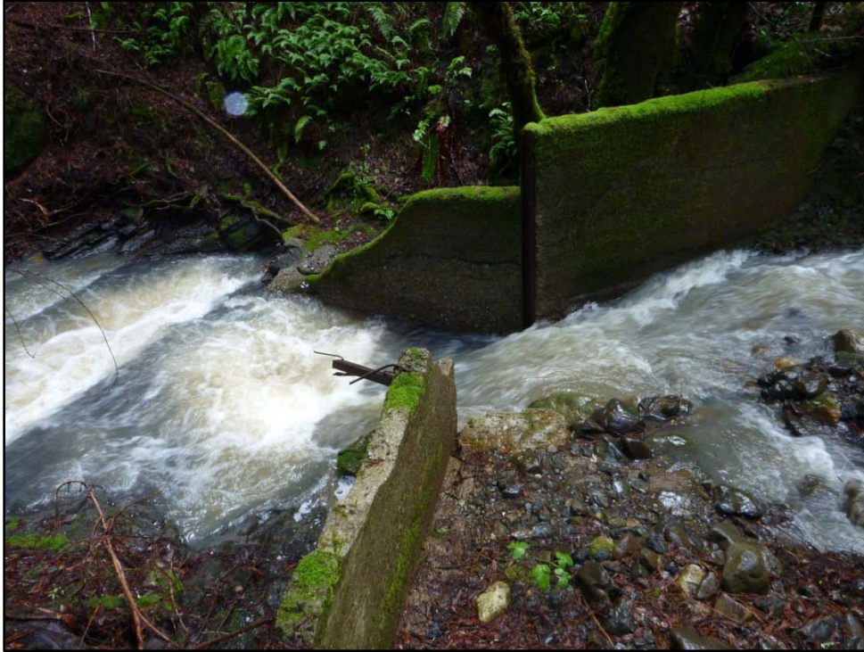
Figure 3. Defunct flashboard dam during a winter storm.
