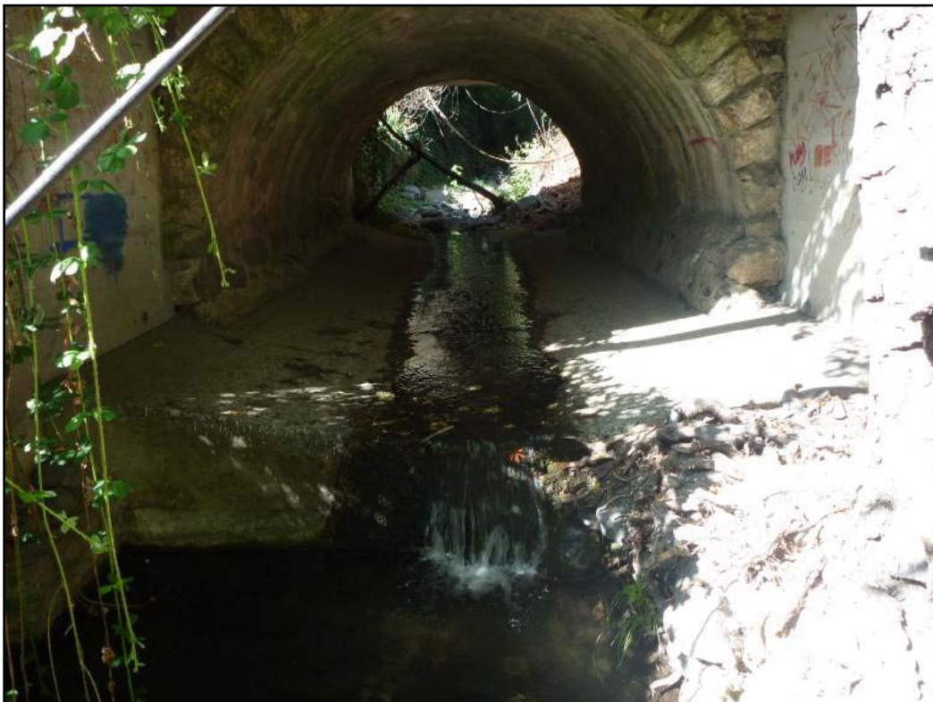
Figure 3. View of downstream end of culvert looking upstream.
