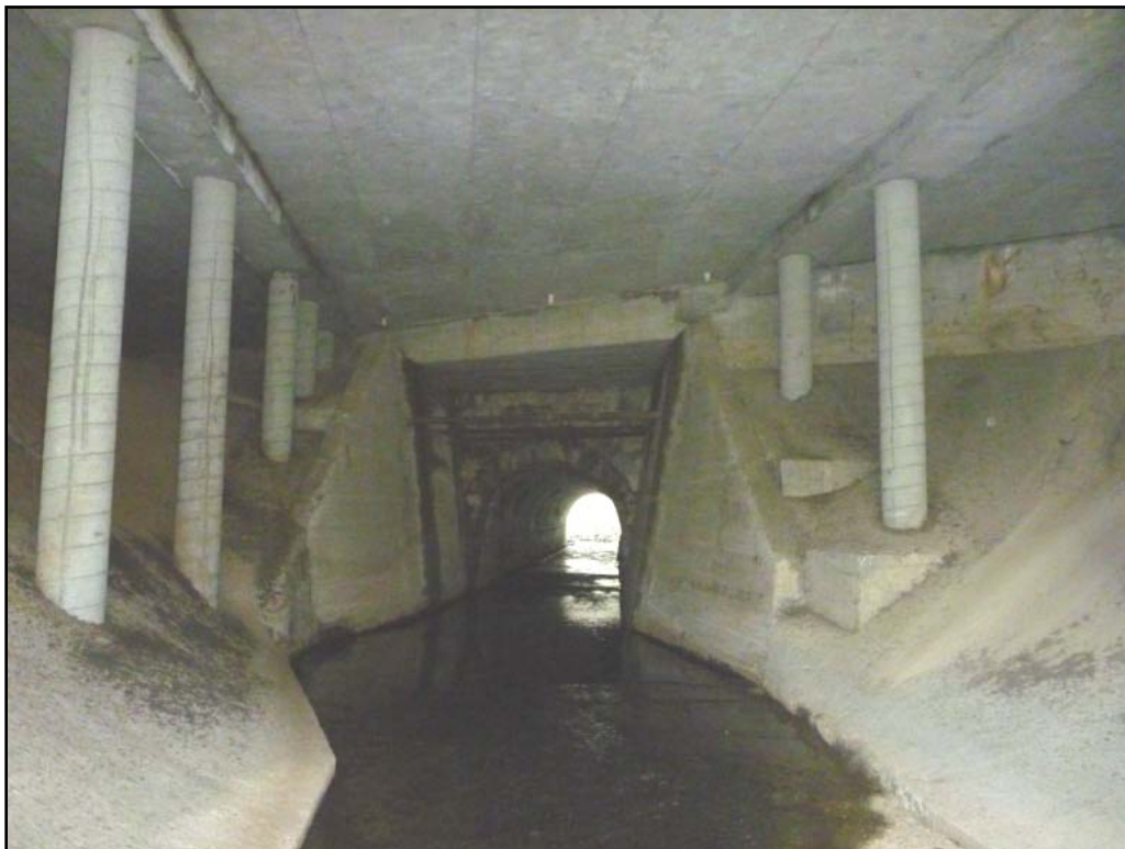
Figure 3. View of box culvert extension and trapezoidal channel looking upstream.
