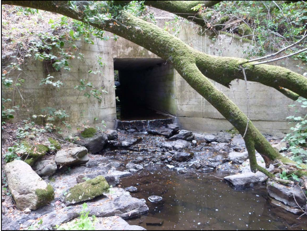
Figure 4. View of culvert outlet looking upstream.
