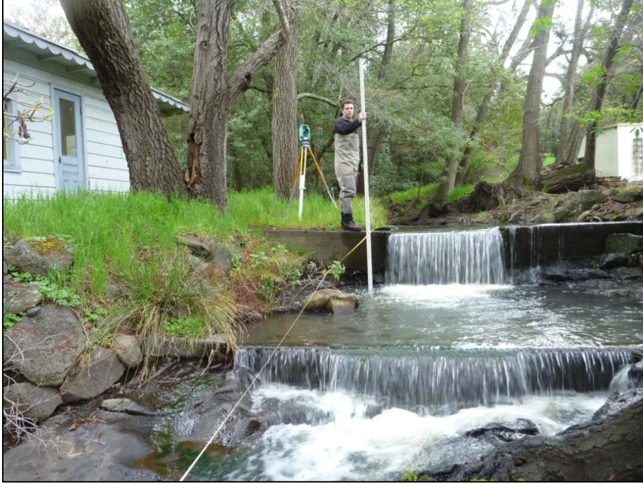
Figure 2. View of the two weirs at site MUR-2 during typical late winter flow conditions (March 10, 2010).
