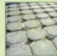
Permeable paving
